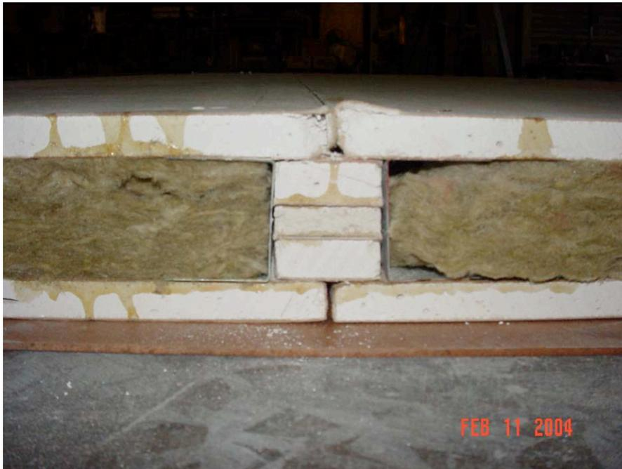
Gypsum filler installed at a panel connection
