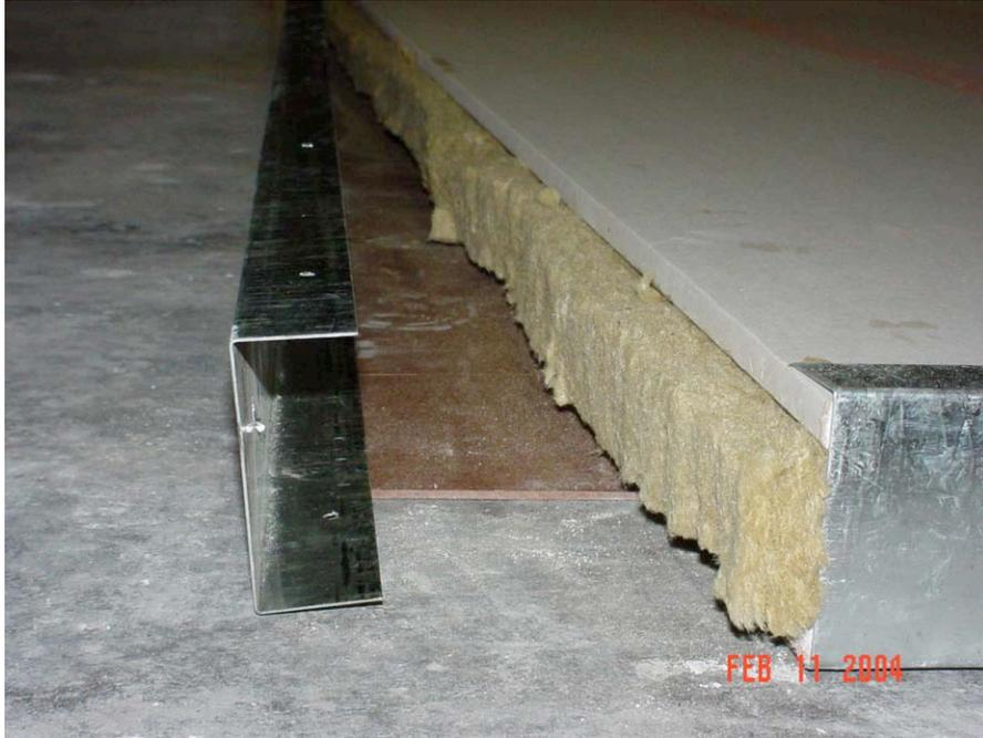
3", 20 GA channel installed around the perimeter
