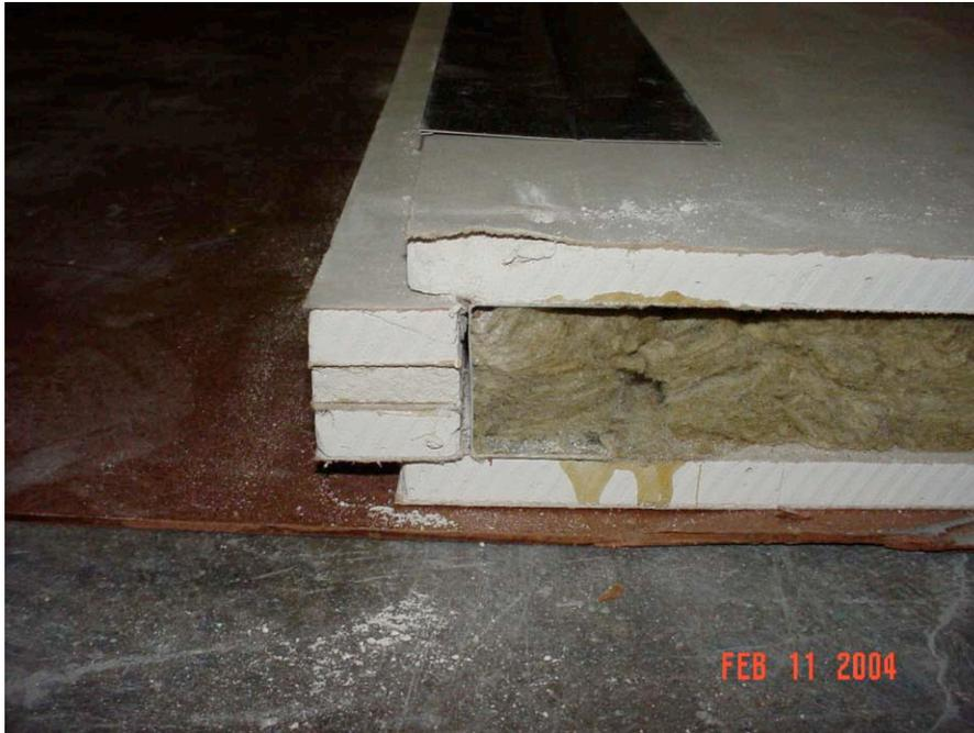
Gypsum filler installed at a panel connection
