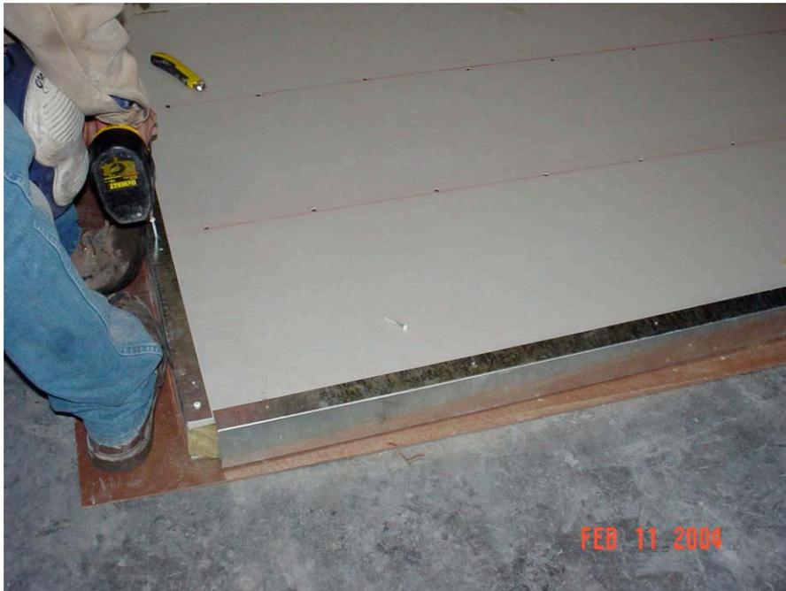
The channel was attached at each stud location with 1-1/2" laminating screws
