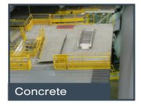
The most durable type of mezzanine flooring by far is concrete. With a high point load and minimal transmission of noise through the deck, concrete should be used in high capacity industrial and military applications where the mezzanine is considered to be permanent. Steel decking is provided with pour stop needed to pour up to a 6-inch concrete floor.
